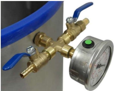
Photo 6: Air manifold correctly installed.
